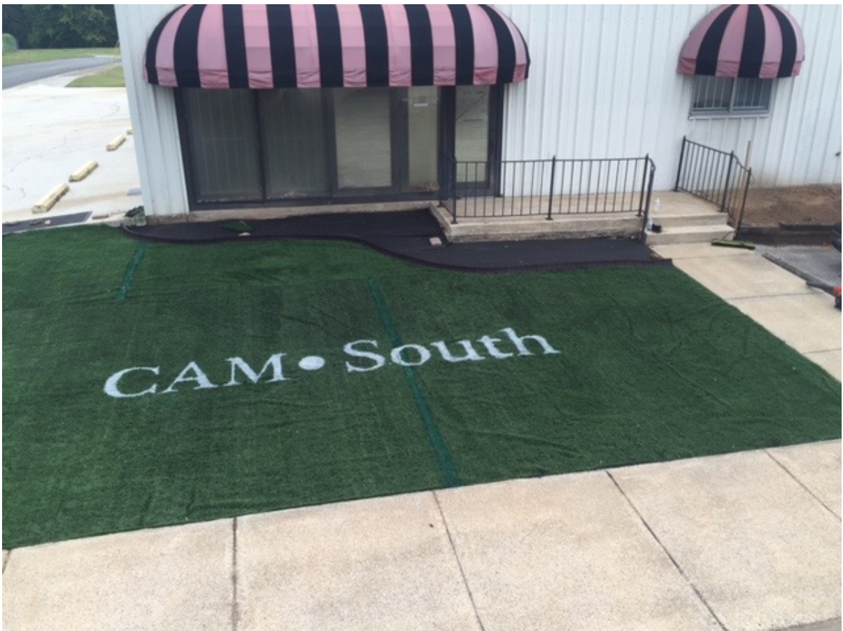
First layer of infill applied, wrinkles are smoothing.
